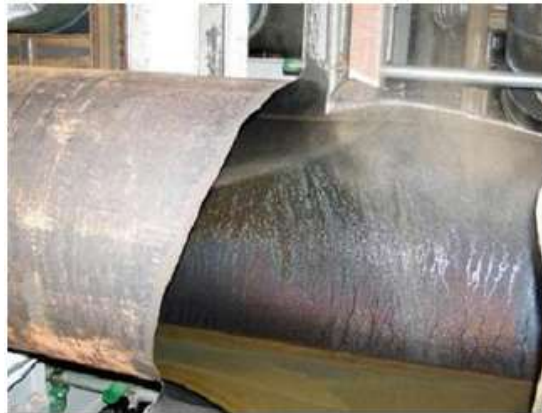
Figure 2. Steam Line Rupture Caused Four Deaths
