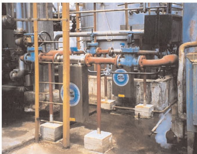
Figure 2. Two parallel D300 sensors on FCC gasoline
