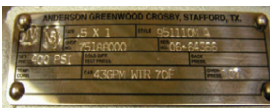
FIGURE 3-12 Typical ASME Section VIII Nameplate
