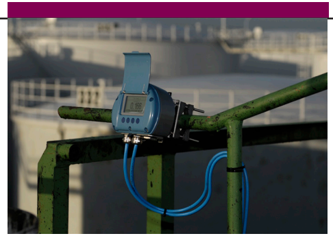
The Rosemount 2230 Graphical Field Display mounted right next to the hand-dipping hatch.
