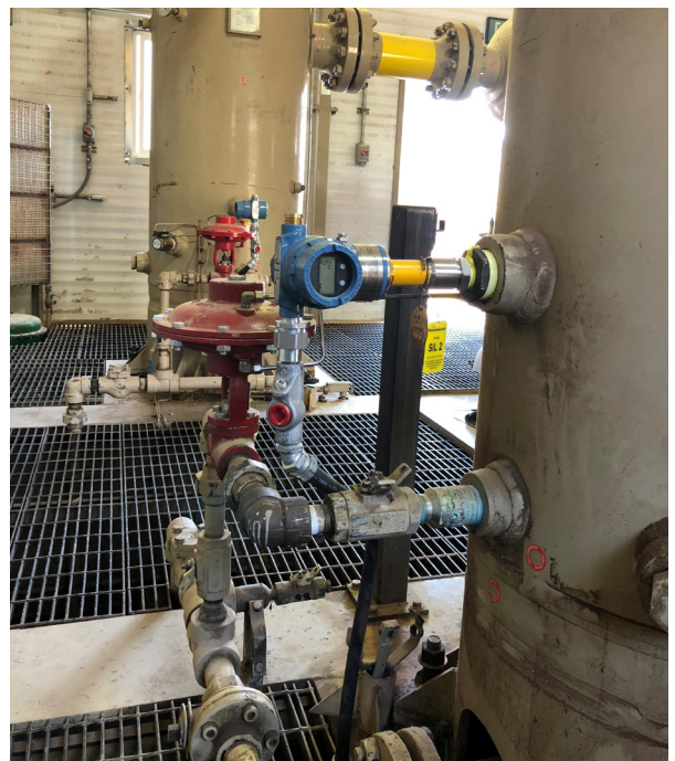
Rosemount 2140:SIS Vibrating Fork Level Detector installed on a scrubber bottle
