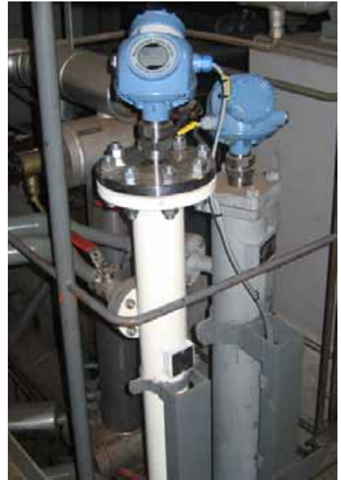
Figure 2. A second Rosemount 5301 replaces the electronic displacer.
