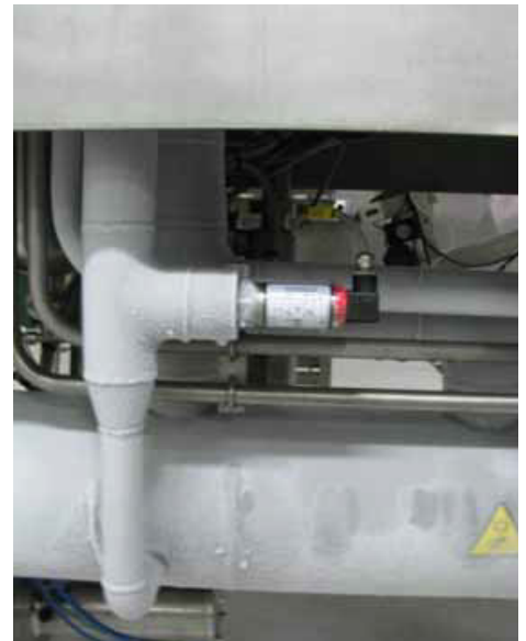
Figure #1: Installed Rosemount™2110 Compact Vibrating Fork Level Switch
