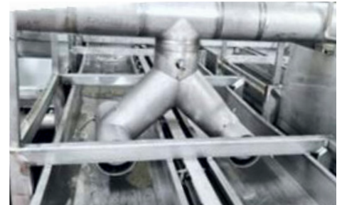
Image 2. Brine sprinkler used on the tanks.
