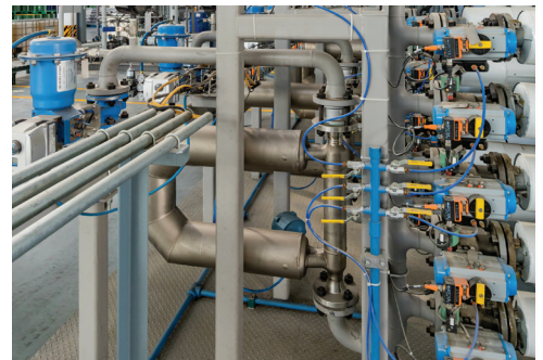
Emerson's In-Line Blenders incorporate our best-in-class Micro Motion® Coriolis flow meters. Photo courtesy of Copton.
