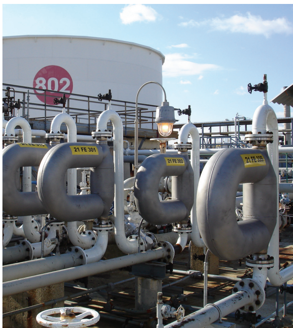
Micro Motion CMF400 blend meters control gasoline blend ratios
