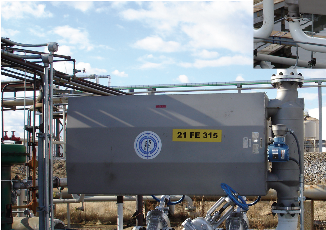
Micro Motion D600 total blend meter measures final product
