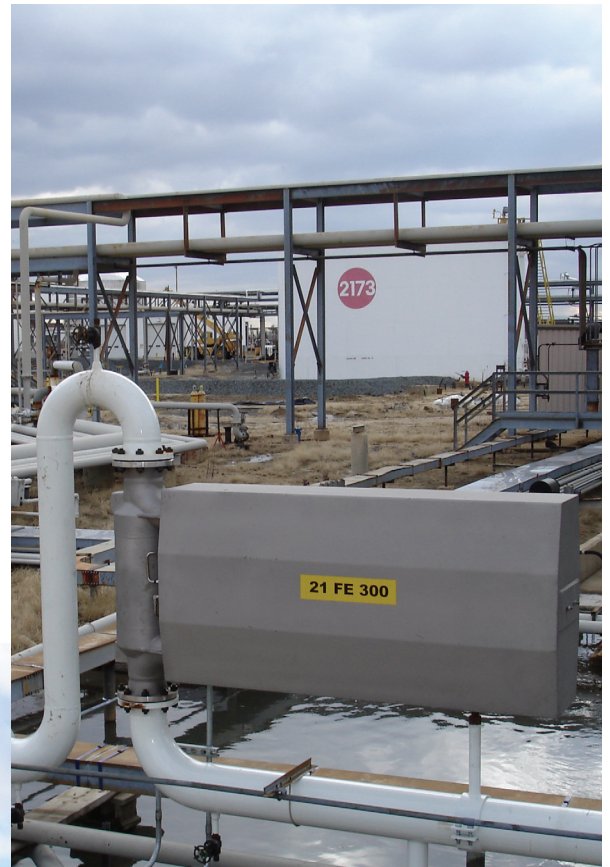
Micro Motion D600 blend meter controls additional component
