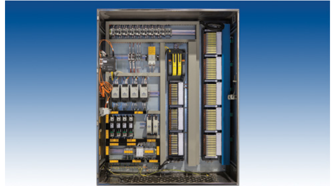
Figure 5: SIS Functional Safety Maintenance and Proof Testing performs much of SIS partial testing automatically.
