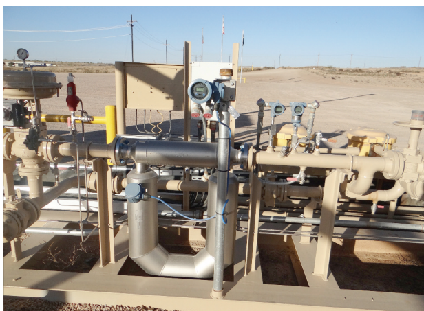
FIGURE 3. An Emerson Elite Coriolis meter is at the core of each load-out point. (Source: Emerson Process Management)
