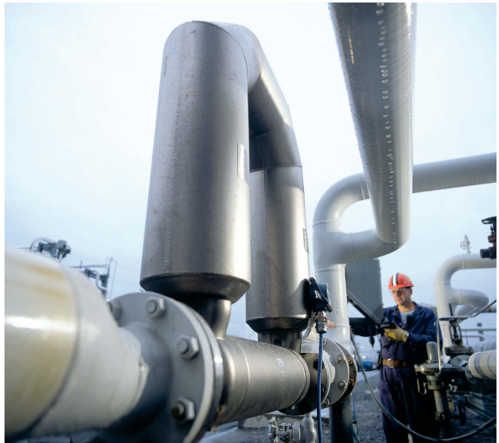
Figure 1: WirelessHART transmitters are used to obtain pressure, level, flow, temperature, and other data from remote facilities, such as offshore platforms and wellheads. All Photo Credit: Emerson Process Management
