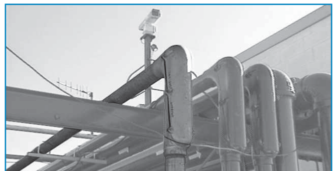
TYPICAL CLASS I, DIVISION 2 RIGID CONDUIT INSTALLATION.
