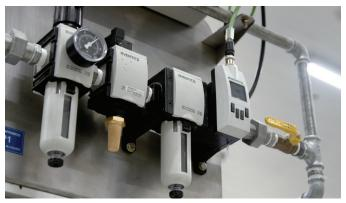
Mounted in-line as a stand-alone device or as part of an air preparation system, the AF2 monitors compressed air usage in real time.
