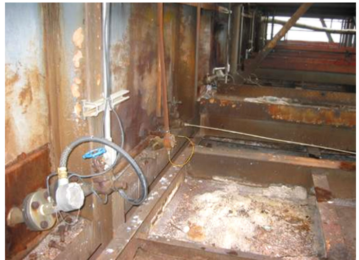
Figure 9 - Four O 2 analyzers placed zone by zone, at the top of the radiant sections.
